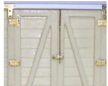
6. Then fit a piece of wire over the door as shown.
