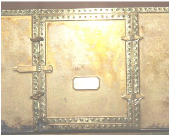
4. Next attach (part 5) the door hinges and (part 6) door latches to the pads on the door as shown. Then attach the door locking bar, which is made from the wire supplied.
